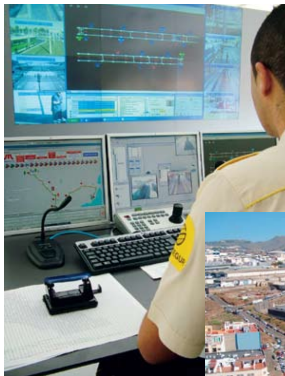
A total of 3 680 solar panels have been installed on the roof of Talleres y Cocheras, which houses the CCP, workshop and depot. The modern control centre is the hub of Metrotenerife operations. Real-time information is displayed on the wall-mounted screen.
